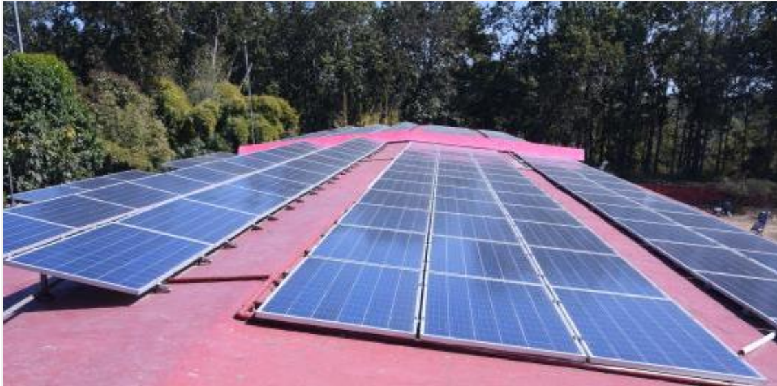
Plate 5: Assessment of the rooftop solar panels in the premises
